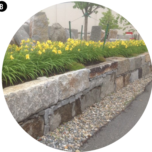
QUARRY BLOCK RETAINING WALL/BENCH
