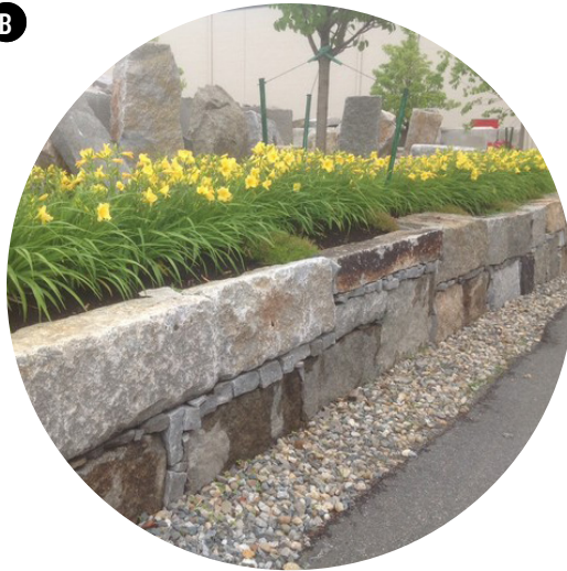
QUARRY BLOCK RETAINING WALL/BENCH
