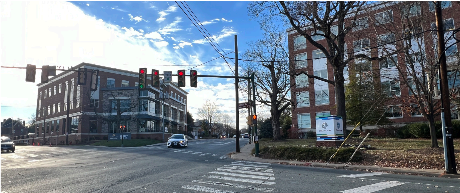
09 | 3-story Urgent Care Facility
