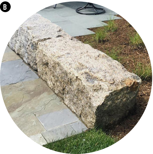
QUARRY BLOCK RETAINING WALL/BENCH
