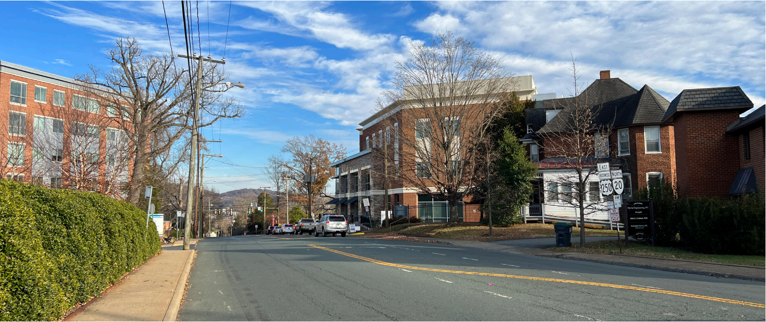
08 | 5-story Office, 3-story Urgent Care Facility, 2 & 2 1/2-story Offices
